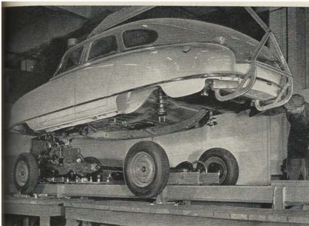
Nash body built as single unit including frame is dropped on what remains of chassis on test assembly line
